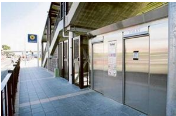
Clean and convenient: A new Exeloo automated public toilet has been installed beside Cabramatta train station as part of the Southern Sydney Freight Line construction deal with Fairfield Council. Picture: Wesley Lonergan
