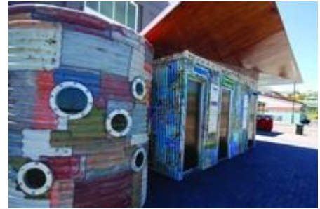
A Helensville public toilet made of corrugated iron sculpted by Jeff Thomson. Photo / Supplied
